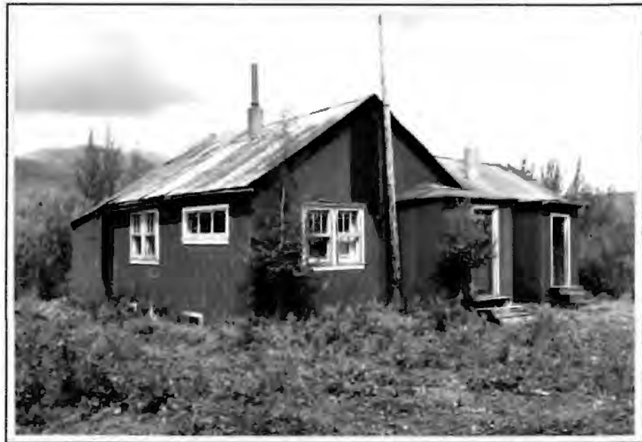
Figure 21. The Alderson House, 1993. The view is looking northwest.
